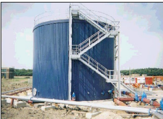
This photo shows a digester complete with cladding and Stair tower
